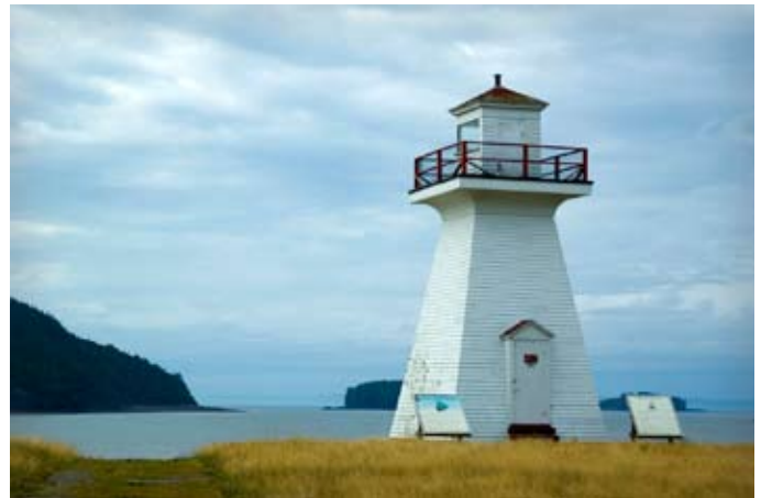
BAY015 - Five Island's Lighthouse
